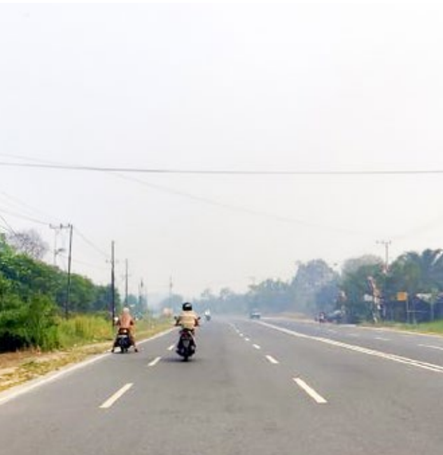
Streets in the Capital of Katingan Regency [Kaltimtimes, 2023]
